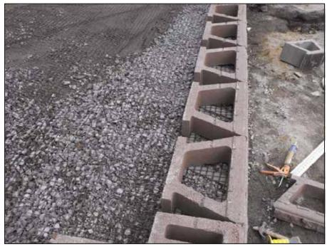
Drainage Aggregate (Inside and behind units)
